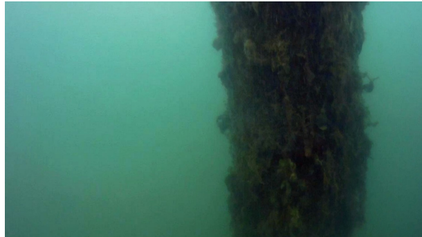
(c) Heavily biofouled lower portion with soft, repetitive algae structures affected by water motion.
